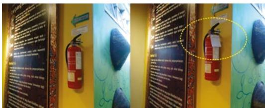
Inclusion of check list cards on fire extinguisher will facilitate the checking, so expect fire extinguisher will be ready to use if needed.
