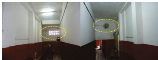
The addition of air circulation in certain spaces, with the installation of ventilation or a fan, aims to make the room cool and not stuffy.
